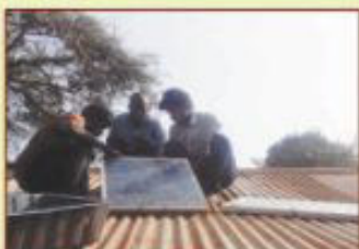
Troubleshooting of Remote Tribal Habitat Solar Light
